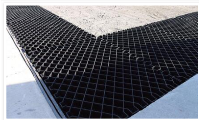
Figure 7 – Diamond Grid™ and expansion joint installation adjacent to Edge Thickening
