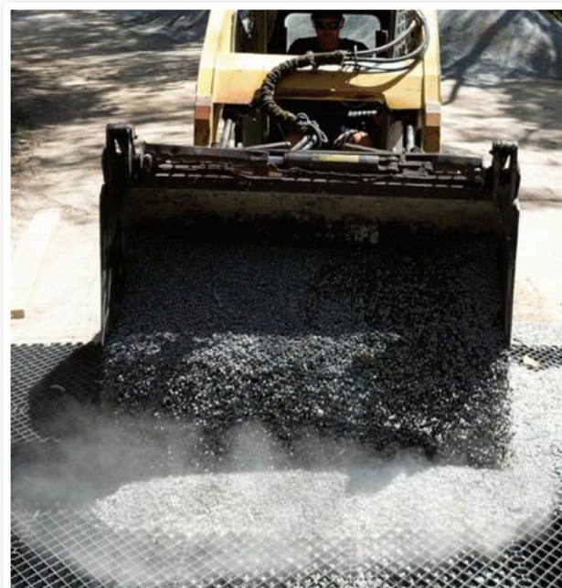
Figure 27 - Filling Diamond Grid with aggregate.
