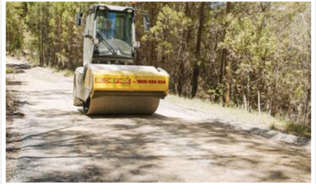
Figure 17 - Subgrade Preparation: Graded and compacted.
