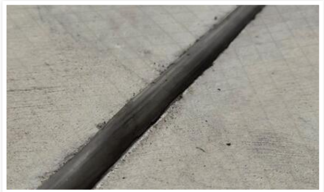
Figure 8 – Seal edges with a trafficable adhesive sealant after pouring to prevent water ingress.
