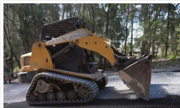
Figure 28 - Utilizing a skid steer (ideally with a spreader bar) to efficiently infill Diamond Grid.
