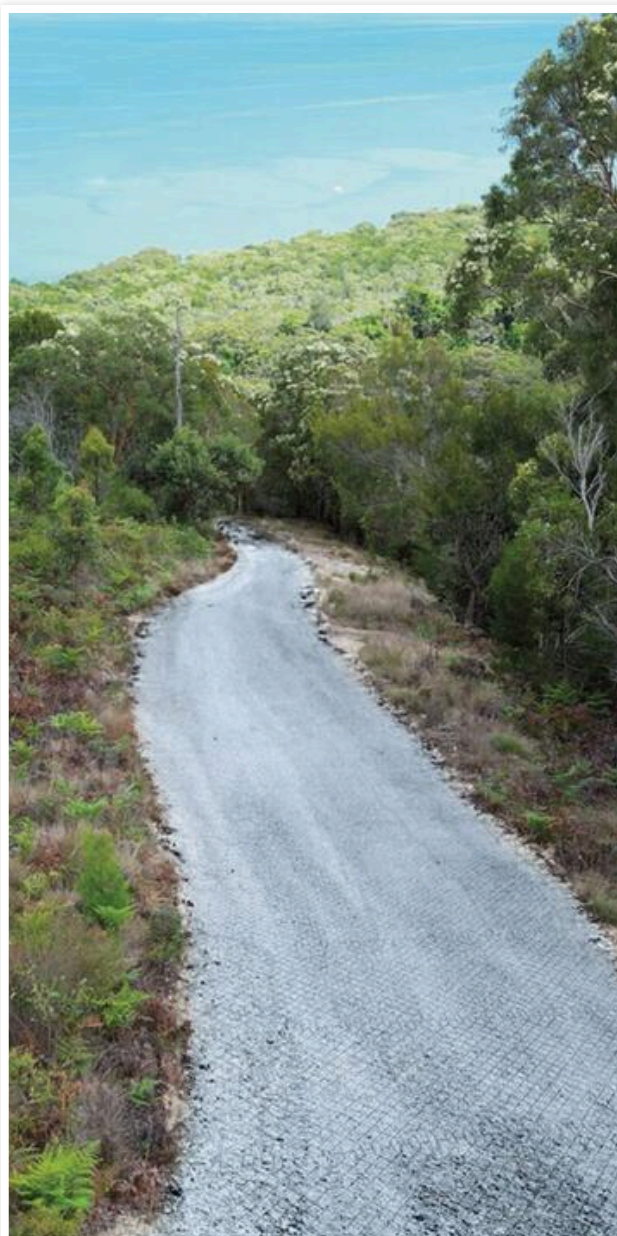
Figure 31 - Completed Diamond Grid™ permeable unbound pavement.
