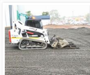
Figure 4 – Subbase Preparation: Spreading and leveling road base prior to compaction. Compacted and watered, ready for Diamond Grid™ installation
