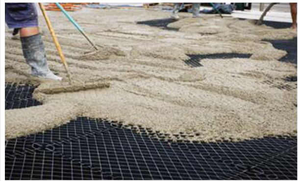
Figure 13- Concrete mix should be approx 180 slump 5 – 7mm stone up to 10mm for Easy Pouring into Diamond Grid™
