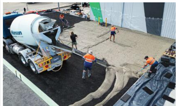
Figure 14 - Spread concrete evenly over Diamond Grid, filling all spaces by hand with rakes and squeegees or vibrating screed for larger projects.
