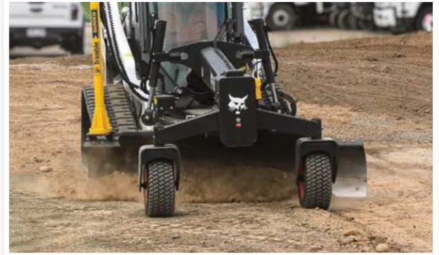
Figure 1 – Subgrade Preparation: Graded Prior to compaction and levelling.
