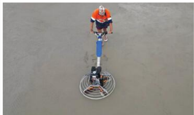
Figure 16: Concrete finishing work in sections, using a trowel machine.
